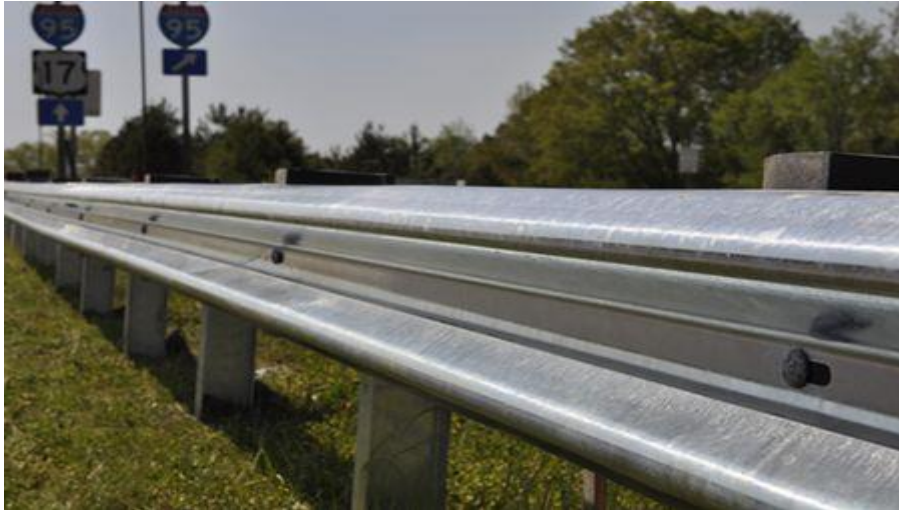
Figure 2- 2. W-Beam Steel Safety Barrier (Semi-Rigid)
