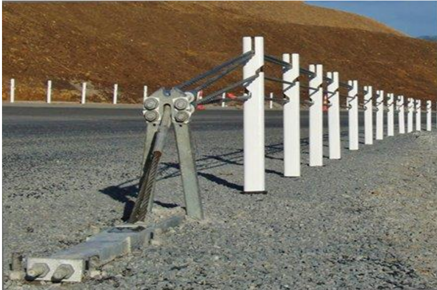
Figure 2- 3. High-Tension Cable Barrier at Posts End (Flexible)
